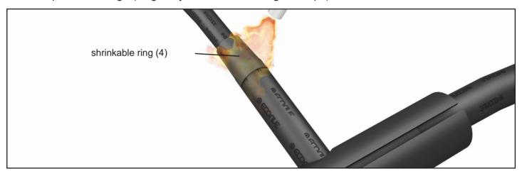
5) Then, continue with the application of the closure patch on the band previously wrapped and start the heating phase up to complete heat-shrinking and sealing of the stretch on the line pipe.
